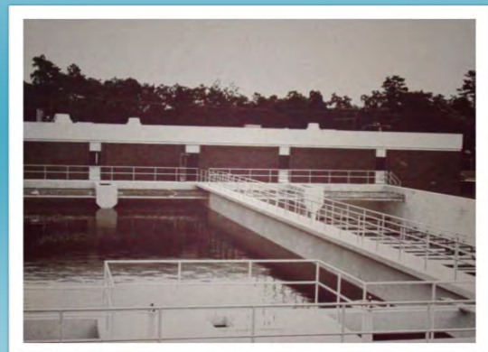
Surface water treatment plant at Brick Township MUA (circa 1987)
